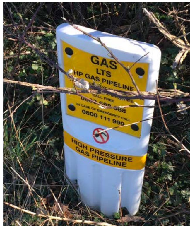
Gas pipeline marker
