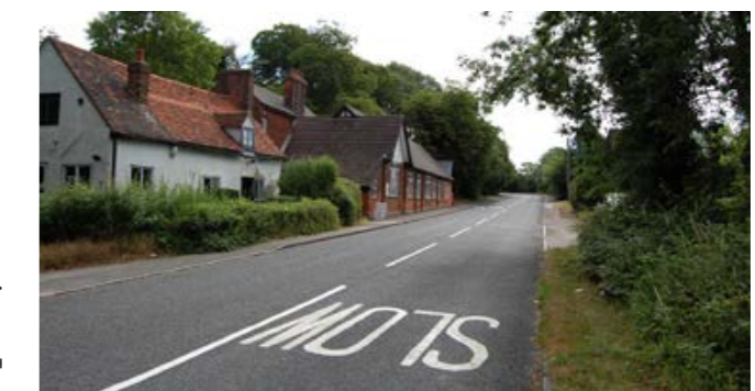
Looking east along Vicarage Lane West, with church and associated buildings on the left (view 4)
